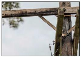
dispatch a line crew to patrol a specific portion of the circuit. There the crew identified the cause of the problem, a line conductor displaced from its normal position on an insulator and lying on its wooden crossarm. As shown in the photograph above, the crossarm had substantial charring.
