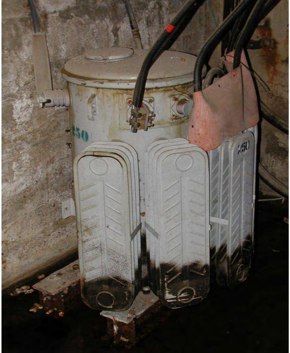
Cortland vault leaking transformer
