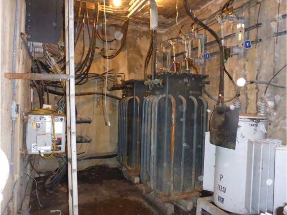
Vermeulens Vault with live front transformers and live front facing fuses
