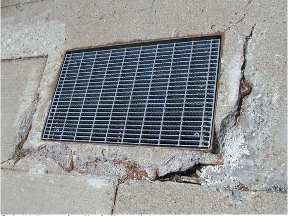
Cortland Vault entrance from sidewalk with exposed rebar
