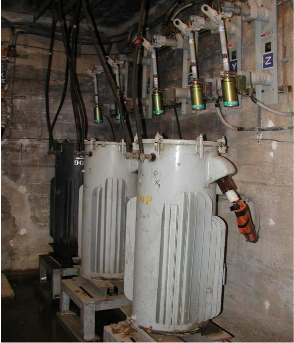
Cortland Vault with live front transformers and fusing
