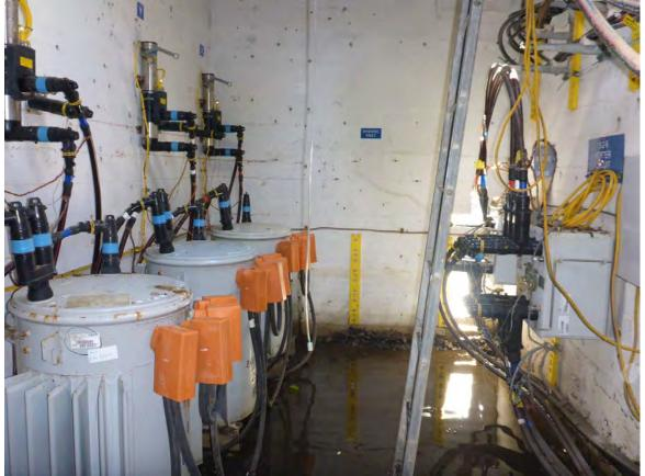
An example of new standard metro electrical equipment, including dead-front transofrmers, dead-front disconnect switches, and SF6 switches, in the Masonic Vault
