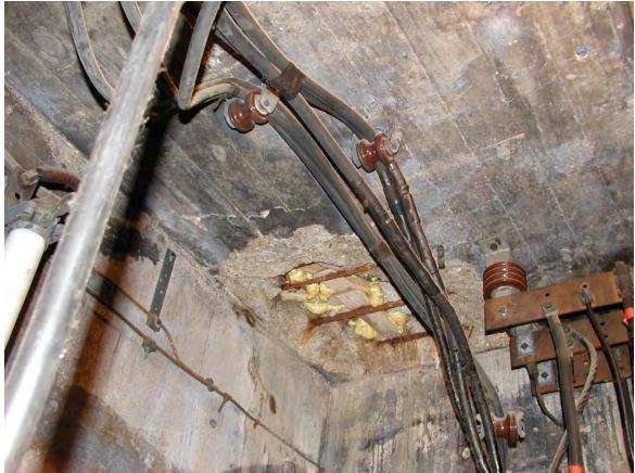
Otsego Vault secondary connection bus bar hanging from ceiling next to hole in sidewalk patched by wood and expanding foam
