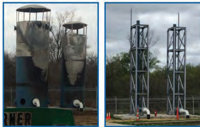
Figure 2. Old and new straight pipe designs
