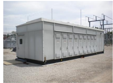
Two-Tier Switchgear
