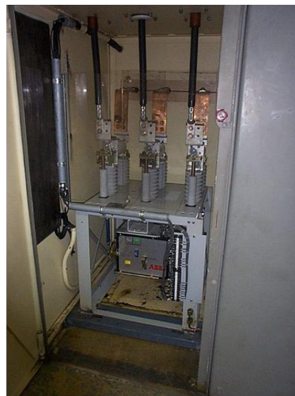
Modern Distribution Vacuum Breakers
