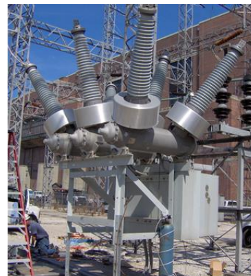
Modern 120 kV Gas Breakers
