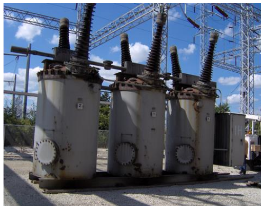
Traditional 120 kV Oil Breakers
