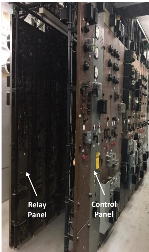
Old Marble Relay Panel (Separate panels for relay and control functions)
