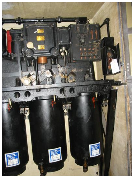
Traditional 4.8 kV Oil Breakers
