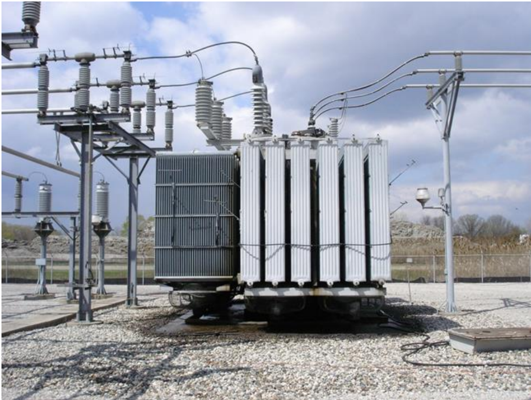
Exhibit 4.1.1 Substation Power Transformer
