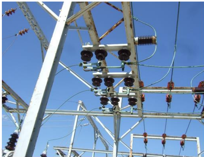
Exhibit 4.4.1 Cap & Pin Disconnect Switch
