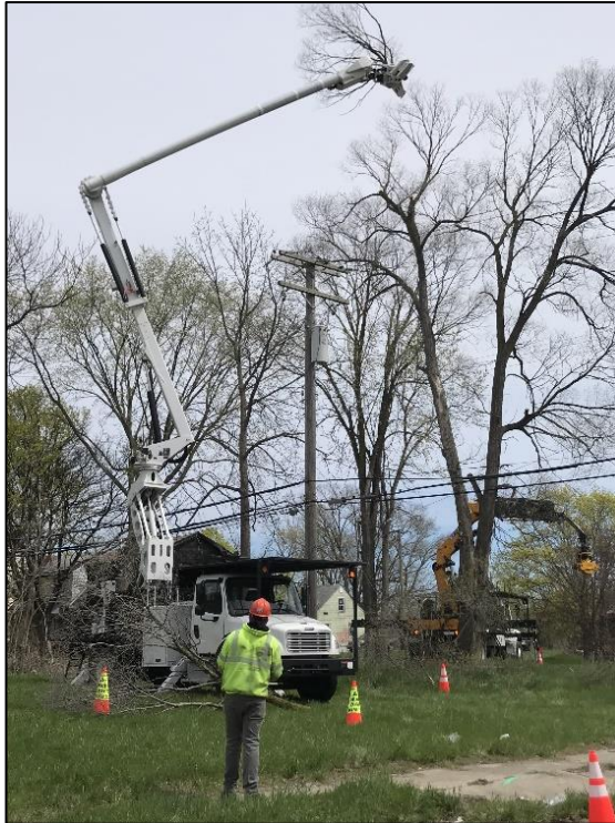
Image 3 Insulated Boom-Mounted Saw
